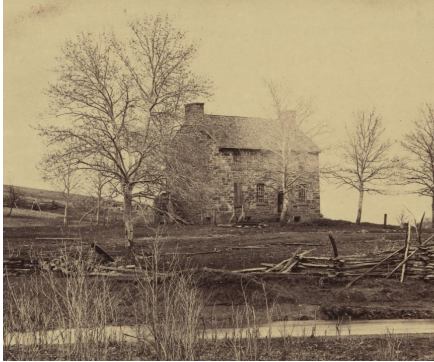
Figure 11 Mathews House, now Stone House
