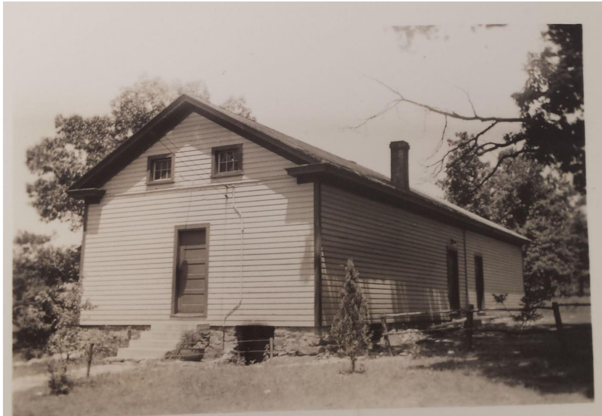
Figure 1 Willisville. Notice barred window at dirt level. This was the coal room.
