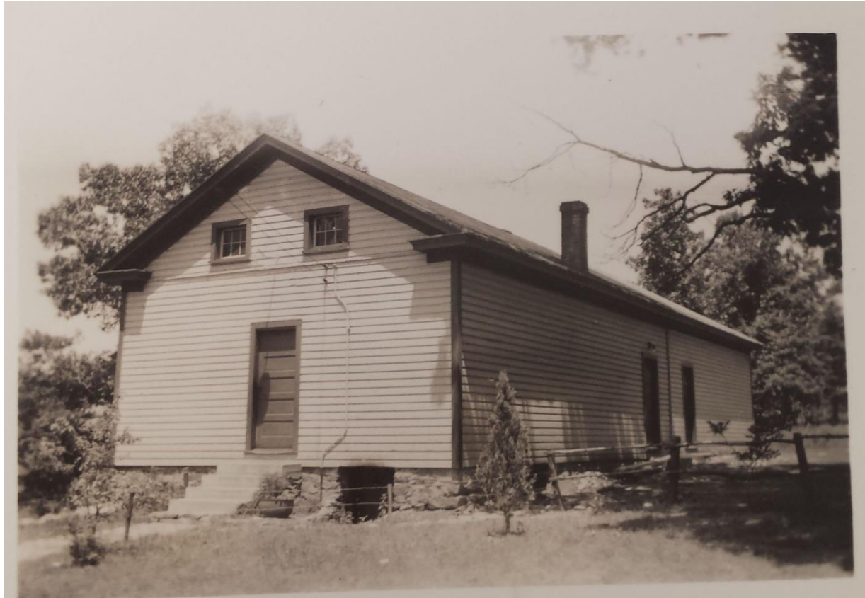
Figure 1 Willisville. Notice barred window at dirt level. This was the coal room.
