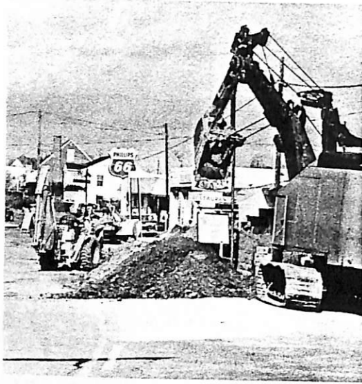
1970. Laying lines for Lovettsville's water and sewer system.
