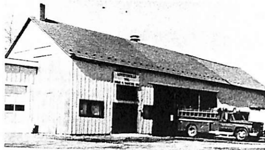
Lovettsville's first fire house, a former feed store much in need of repair. Members of the Fire & Rescue Company did the work of renovation themselves.
