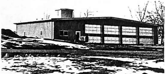
New Fire House recently constructed and in use.
