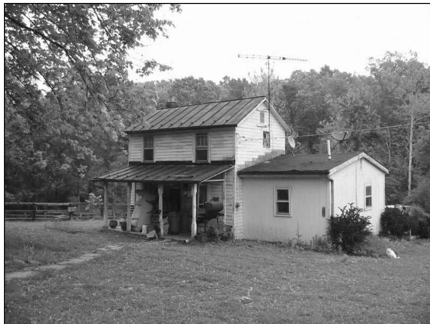
Figure 16. House, 20058 Sycolin Road, Sycolin. Façade or west elevation (DHR #053-5215).
