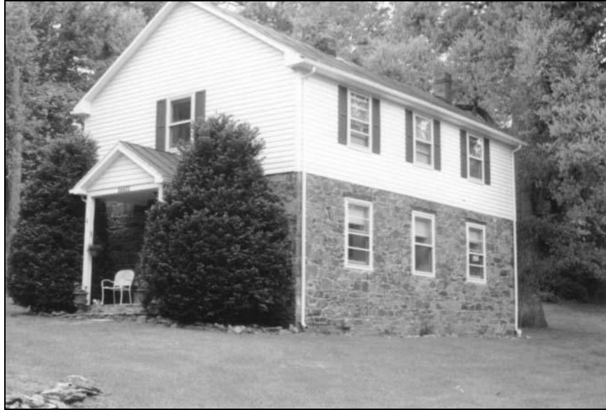
Figure 22. Lincoln “Colored” School. East and north elevations (DHR #053-0845).
