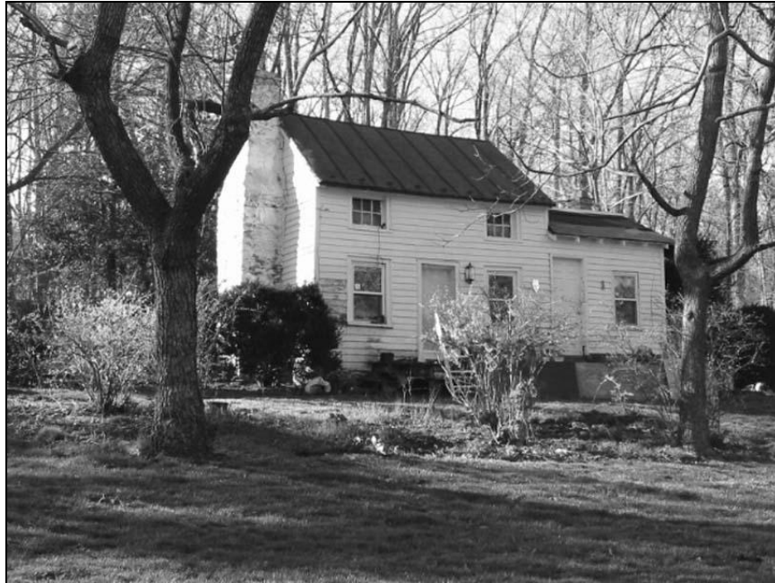
Figure 14. House, 23965 New Mountain Road, Bowmantown. Façade or southeast elevation (DHR #053-0605-0004).
