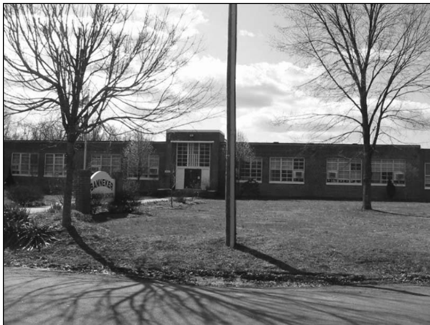
Figure 37. Banneker School, St. Louis. Façade or north elevation (DHR #053-0605-0004).
