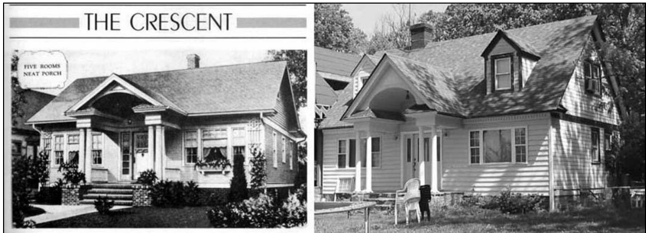
Figure 31. (Right) “The Crescent” Sears House from Houses by Mail by Katherine Cole Stevenson and H. Ward Jandl, John Wiley & Sons: New York, 1986. p.95. (Left) House, 33960 Welbourne Road, Willisville. Façade or south elevation (DHR #053-5116-0011).
