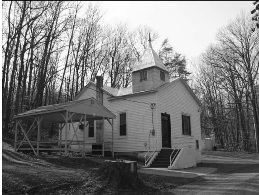
Figure 24. Mount Pleasant Baptist Church, Lucketts. East and north elevations (DHR #053-0322).
