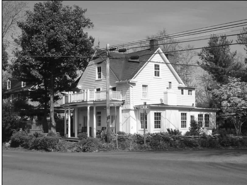
Figure 21. House, 23381 Sam Fred Road, Macsville. South and east elevations (DHR #053-5150).
