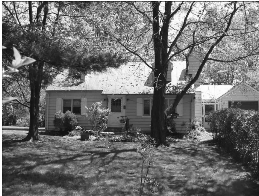
Figure 32. Irene H. Trammell House, St. Louis. Façade or west elevation (DHR #053-5099-0002).
