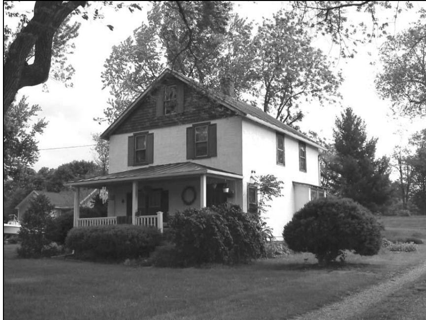
Figure 20. House, 34090 Snickersville Turnpike, Murphy's Corner. East and north elevations (DHR #053-5141-0003).
