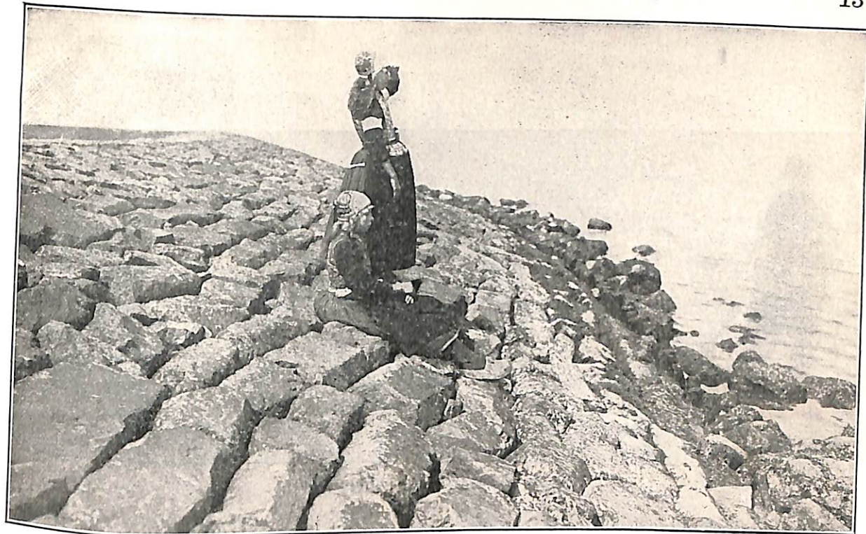
Fig. A. "What a job," you say, "to fit all these big boulders into this dike!" The thrifty Dutch people did it, however, to keep the sea from their fertile land.
