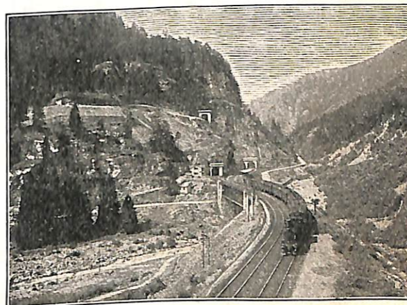
Fig. B. A tunnel entrance on a double-track Swiss railroad. Is there a wagon road in this picture?
