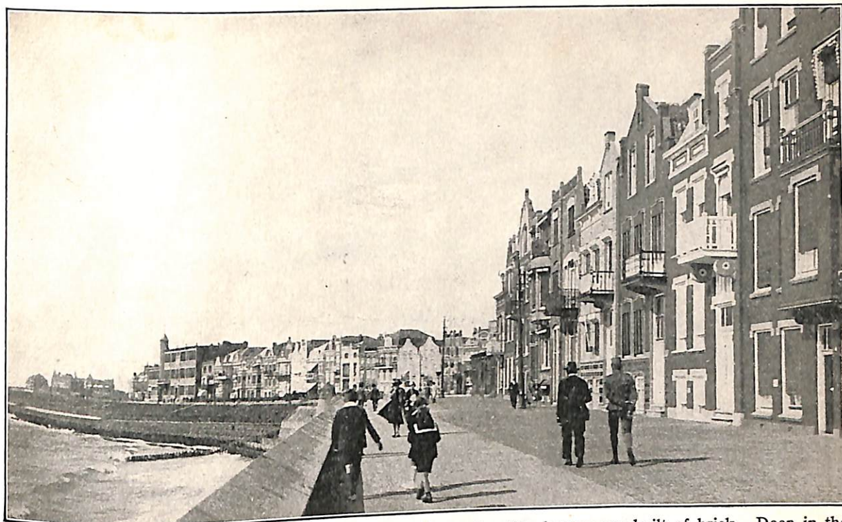
Fig. A. The city of Flushing, Holland, and its stone sea wall. The houses are built of brick. Deep in the ground beneath the wall are rows of piles. They give a firm foundation in the soft mud.
