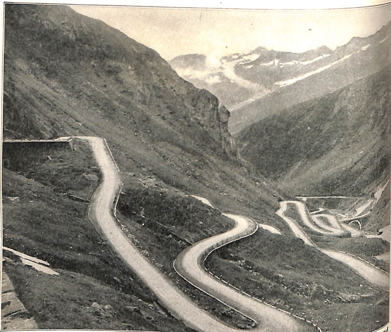
Fig. A. This picture shows a section of the famous St. Gothard Pass in Switzerland. The road winds round and round as it climbs the mountain, in order to avoid steep grades.
