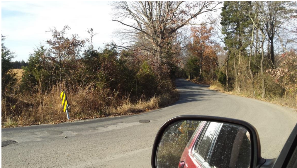
Figure 5 Difficult Corner Looking N along Ticonderoga towards Braddock.
